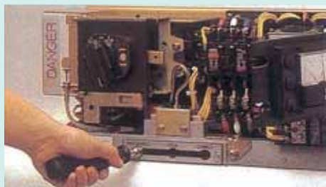
Disconnecting position Inserted the operating lever
