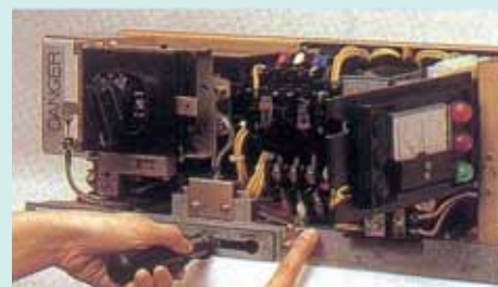
Moving the operating lever toward the right while releasing the operating lever stopper
