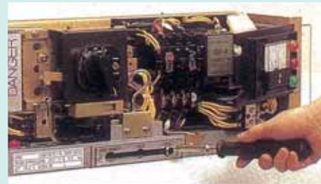
Removing the operating lever
