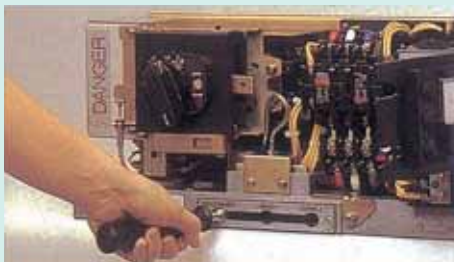
Releasing the mechanical lock at the disconnecting position by complete insertion of the lock collar
