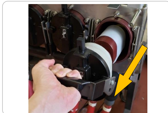
Figure 33. Holder withdrawal (③)
